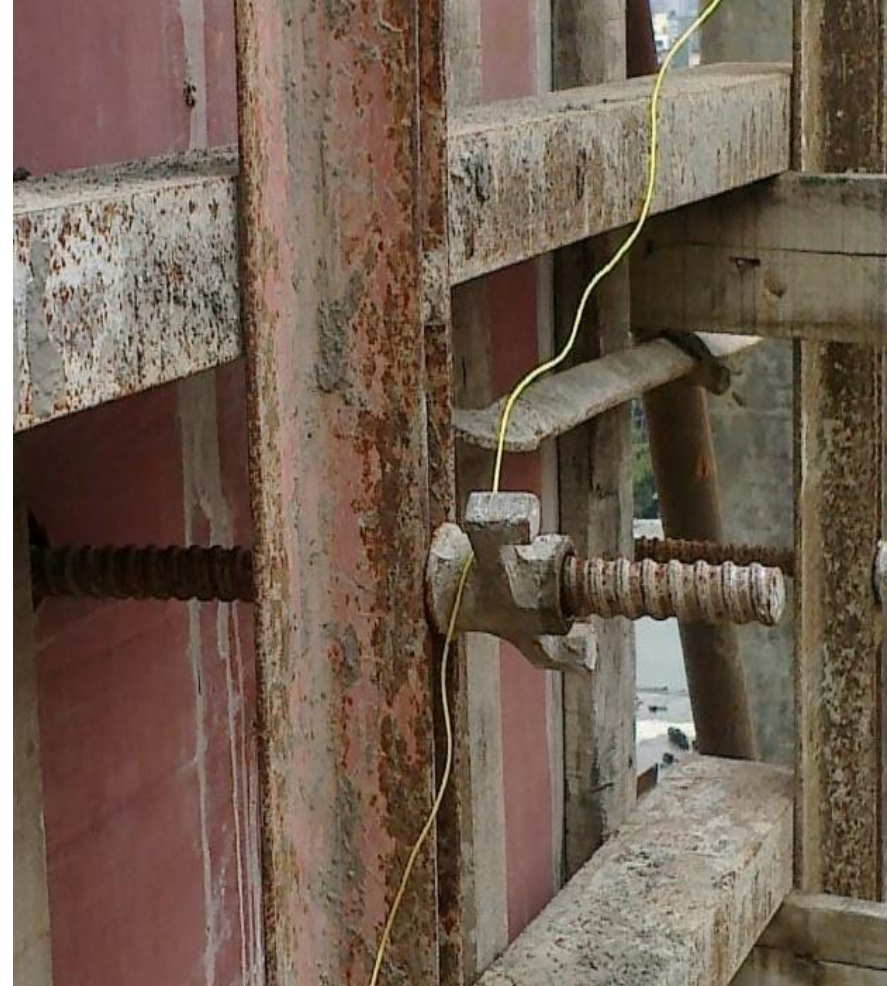
Tie rod in place
