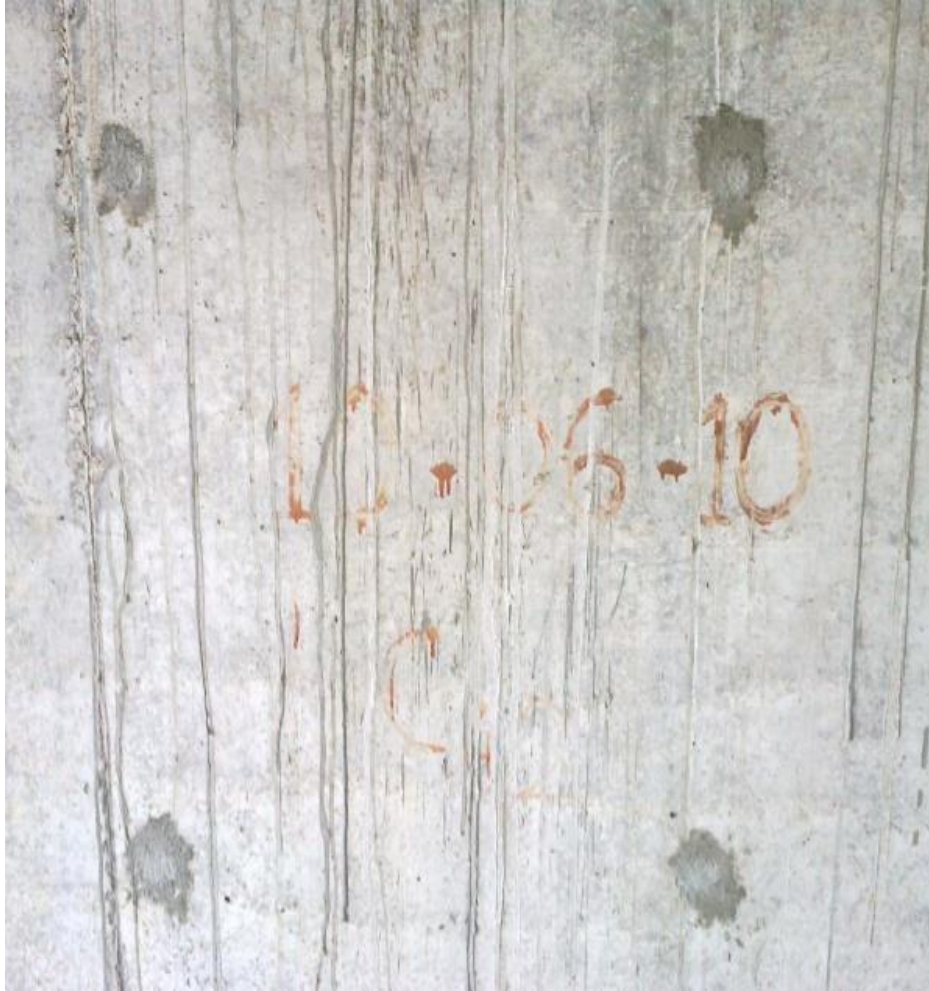
Sealing of Tie rod holes
