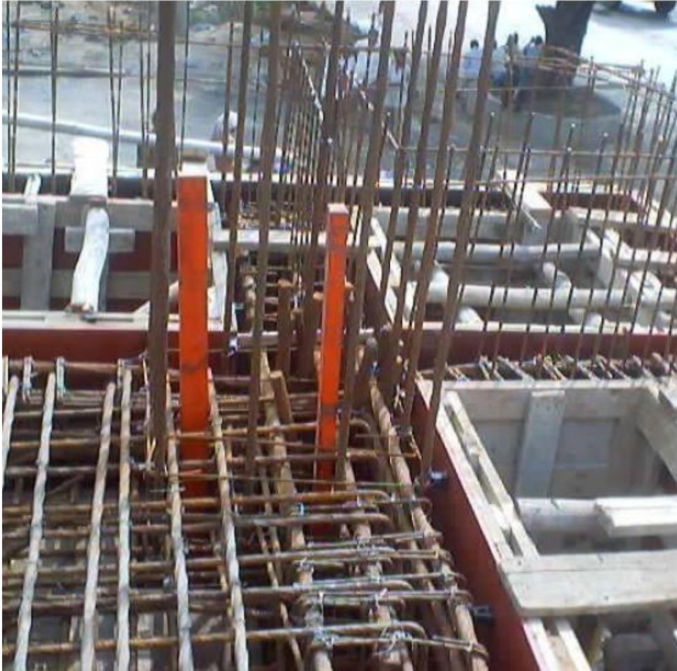
A wooden piece ("Kanda") for column reinforcement during slab casting.
