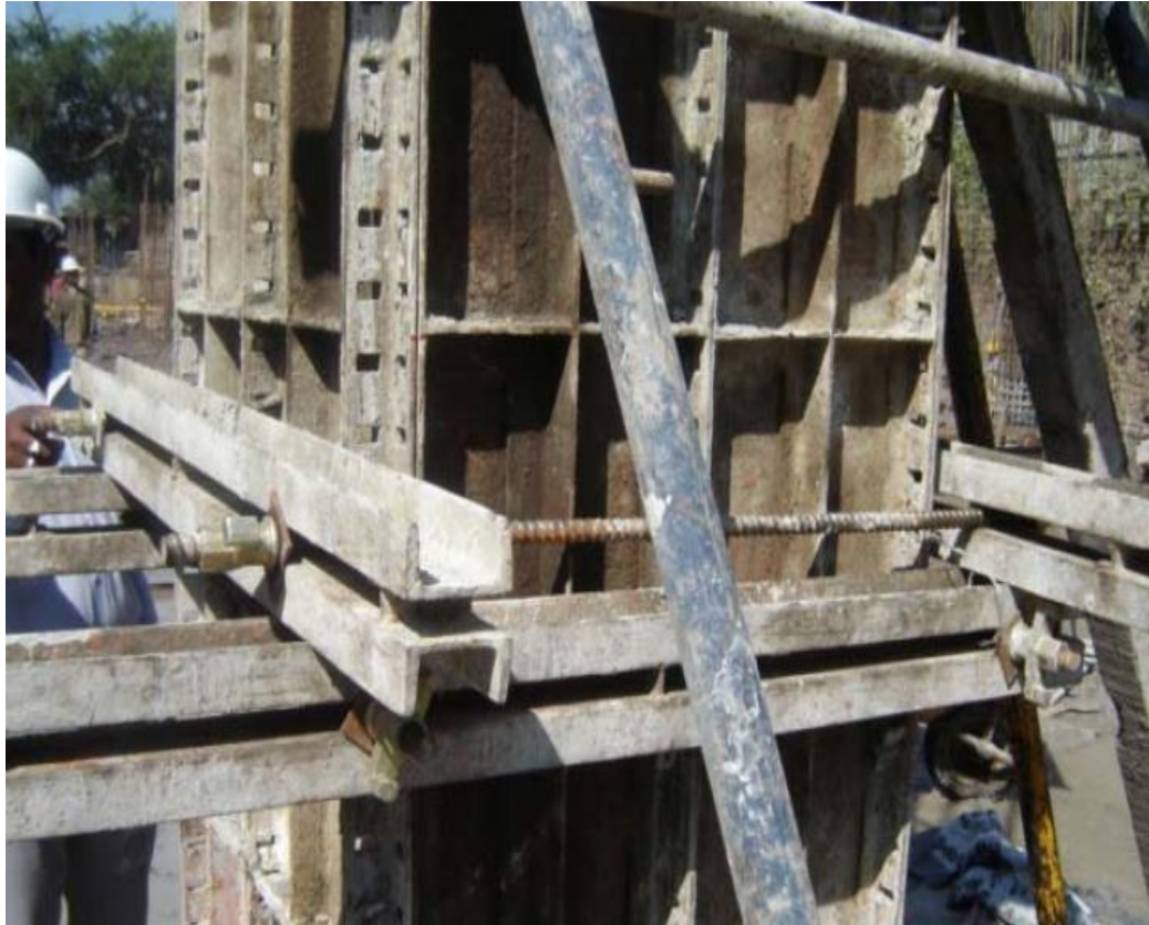
Sturdy shuttering out of steel plates & soldier for columns.
